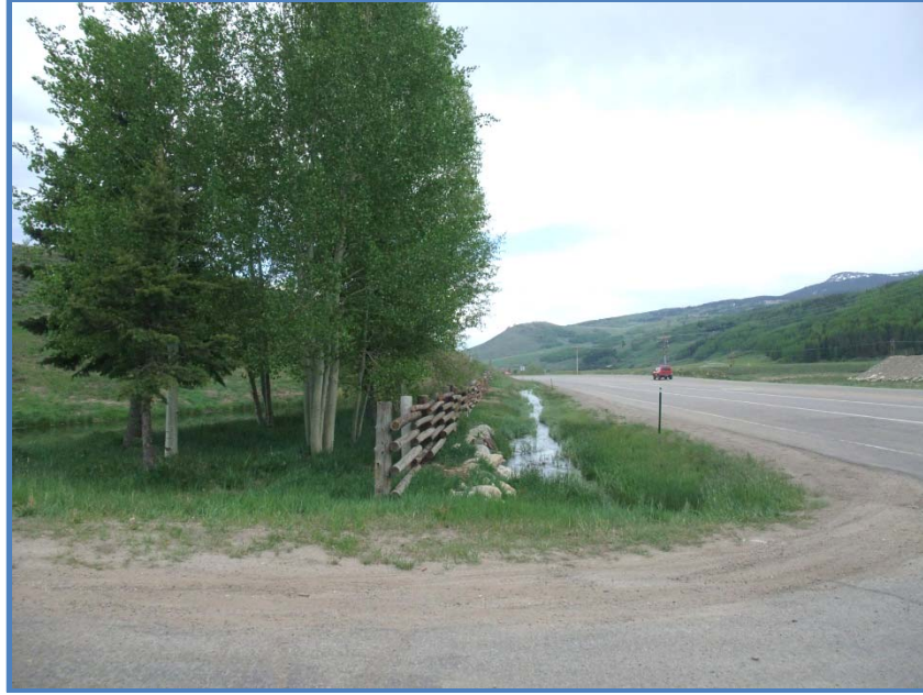
Figure 4 – Buckley Drive (Looking North)
